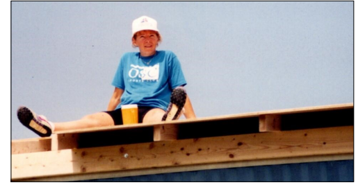
And replaces a roof
